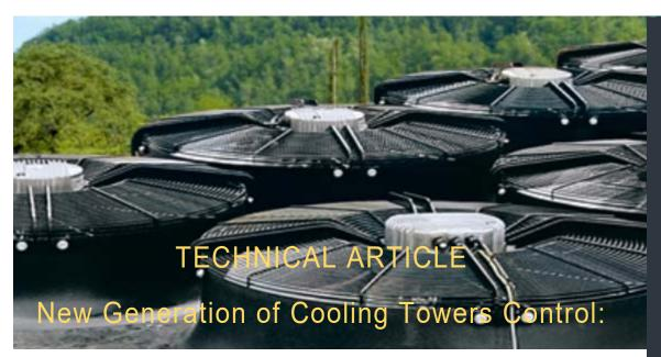
EC (Electronically Commutated) motors are permanent magnet motors which are running on high voltage direct current (DC) electricity with built in AC to DC conversion allowing them to run direct from single phase or three phase mains supplies. They are more efficient, quieter and more reliable compared to AC motors.
